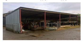
H) Steel portal framed cubicle building, 120' x 36' providing cubicle housing for 60, fibre cement roof cladding, mass concrete walls to 1/3 height and spaceboarding above to sides and rear with feed barrier to front under cantilever overhang. Feeding/scraping passage adjacent to sheeted door giving access to slurry store. Internal strip lighting, water supply with concrete base and apron. Full height sheeted doors to both gable ends.
